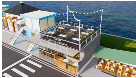
Gambar 9. Coffee Room Lantai 2
